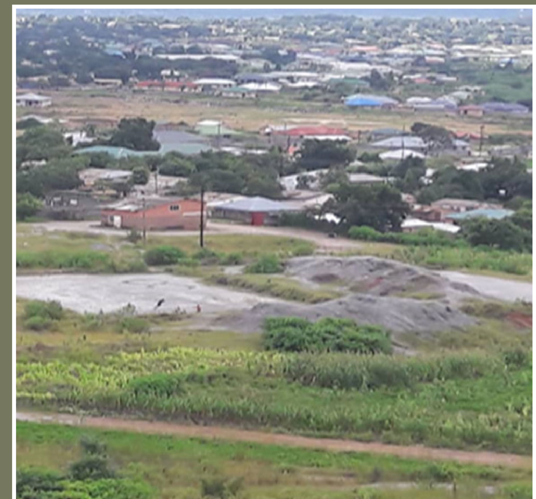
The Waste Rock Dump Inspection Tool.
