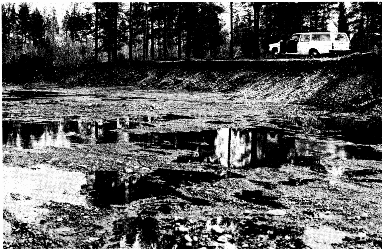
Fig. 84. A shallow excavation in gravel close to station no. 3805. Note groundwater seepage at bottom of excavation. Photo L. Nordberg 1973.
